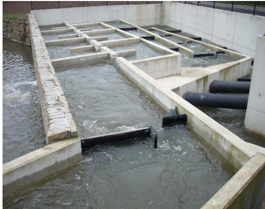
The fish pass of the hydroelectric power plant in Roermond (Netherlands) (Photo: Johan Coeck)
