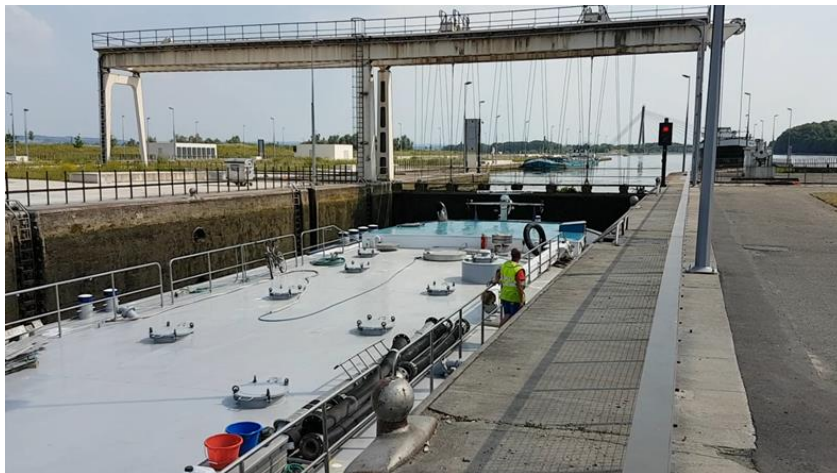
Photo 1: The lock of Lanaye (Wallonia) (Photo: IMC)
