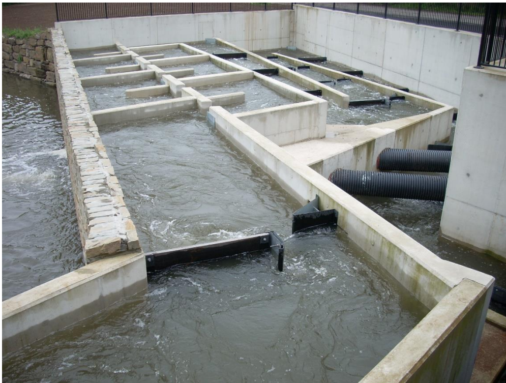
Photo 2: The fish pass of the hydroelectric power plant in Roermond (Netherlands) (Photo: Johan Coeck)
